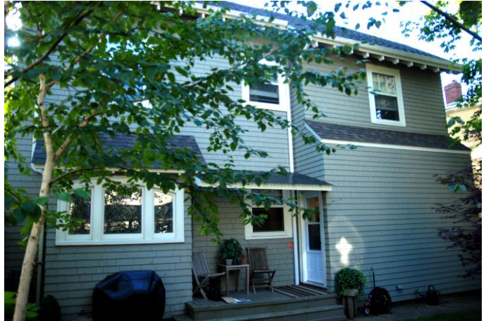
Figure 2: Three-bay building rear including an existing alcove with shed roof extending from the two-storey protruding bay and a historic alcove with shed roof and three ganged stained glass windows.
