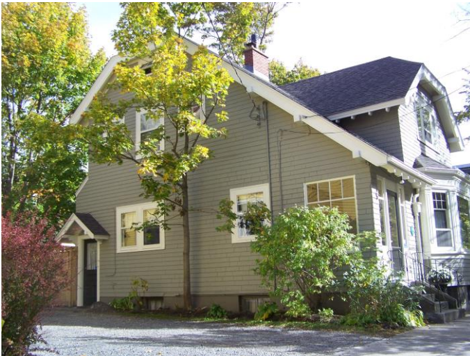
Figure 3: Asymmetric north side elevation including an entryway covered with a gable roof.
