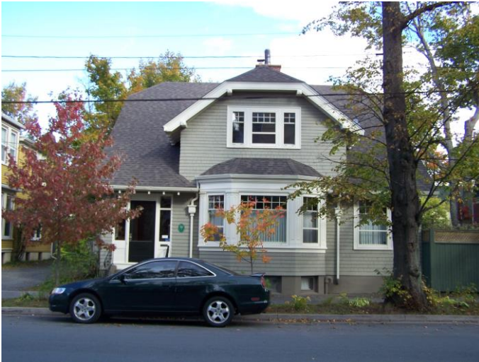
Figure 1: Almost-symmetric front with large hip gable roof, large extended central dormer, and large central bay window (formerly an open porch).
