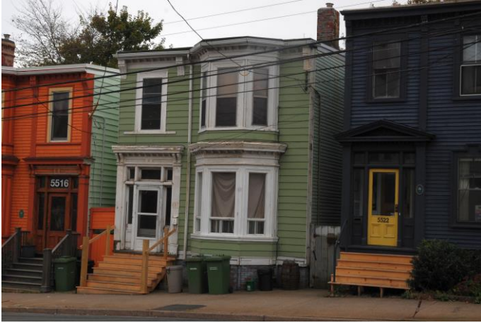
Figure 1: The architectural importance of the building lies in its form as a plain residence of the Late Victorian period with simple box shapes
