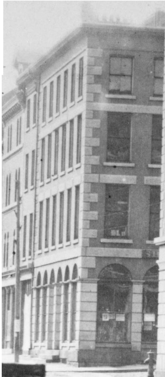
Photo taken in 1871 showing original building including arched windows and frieze/cornice condition
