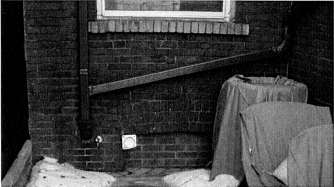
6053 Jubilee Road Rear Elevation Details
