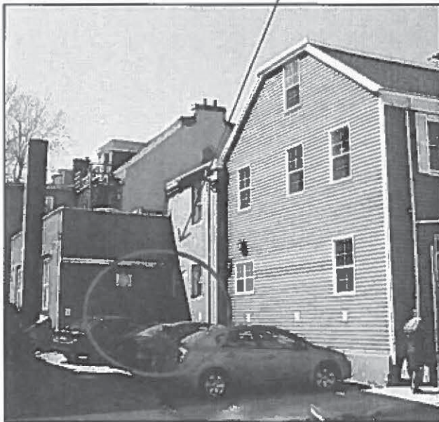
Hollis Street showing rear addition.
