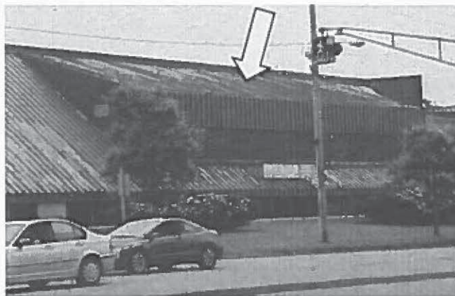
Figure 1. Solar Wall location on top of existing mechanical room
