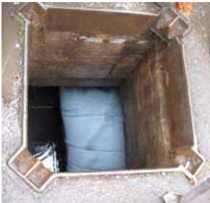
Trenchless pipe liner moving through sewer pipe
