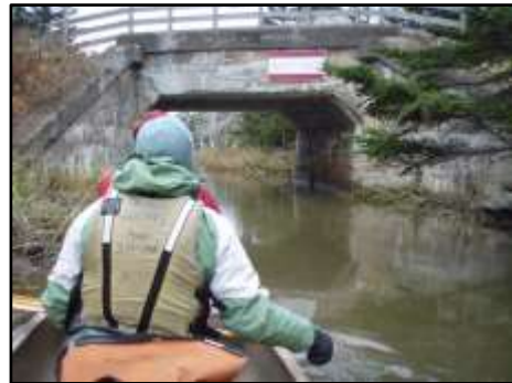
6 Bridge - Atlantic View AT at High Tide
