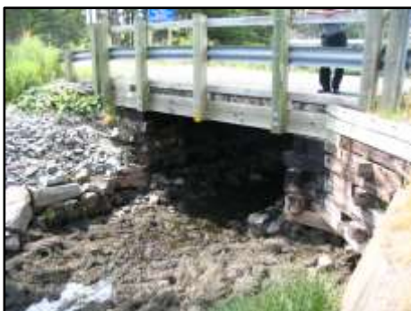
4 Bridge - Highway 207 at Low Tide
