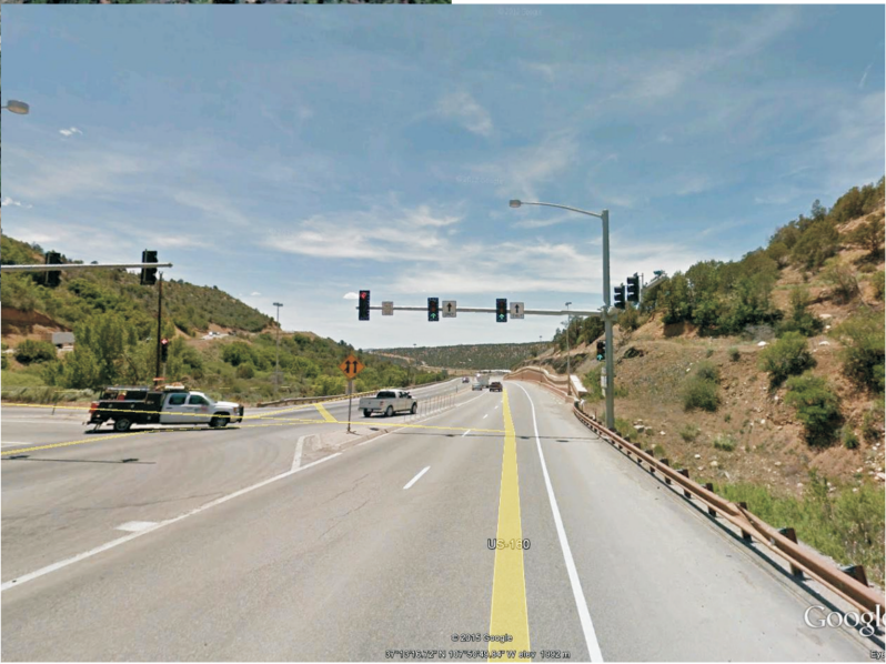
This example intersection near Durango, CO uses delineator posts to separate the left turning traffic from through traffic.
