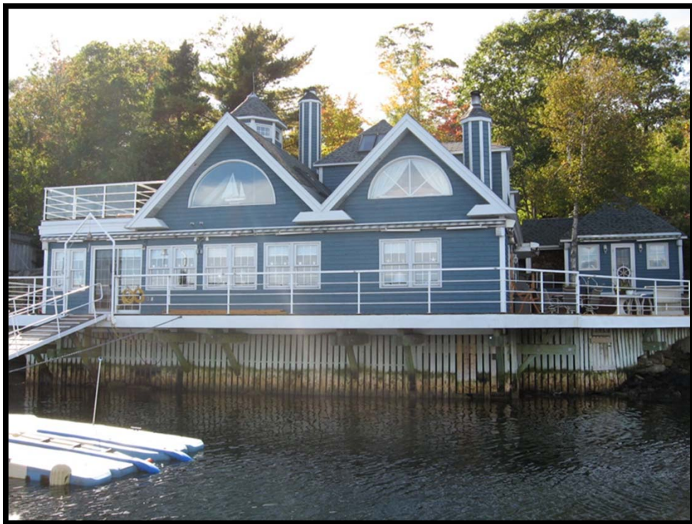
Dwelling on Lot G2 (from dock)
