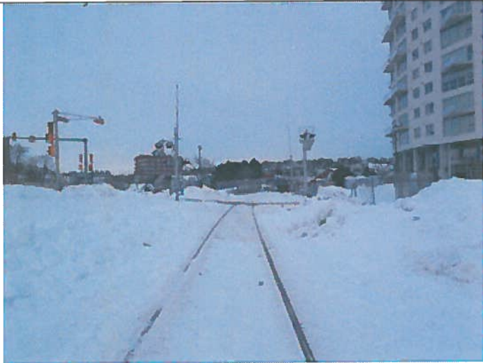
Photo 5: West side of the track, Q looking East
