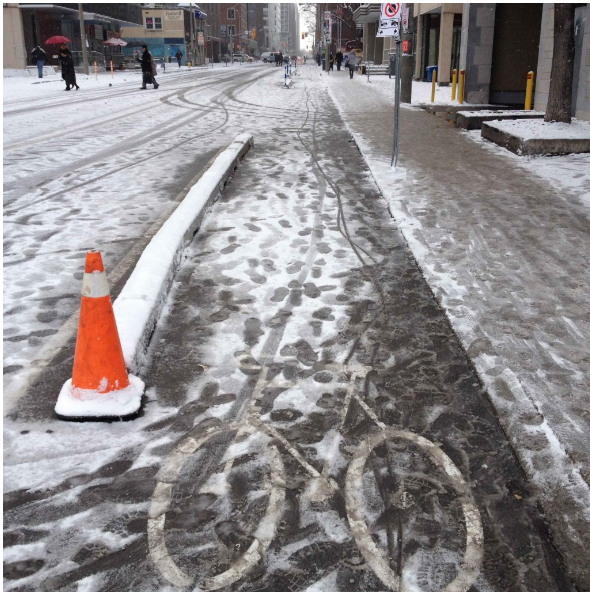
Figure 5-4 Segregated Bike Lane in Ottawa (same condition as roadway and sidewalk)
