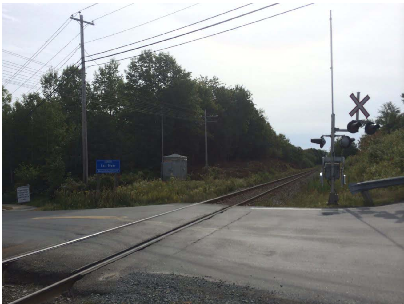
Figure 2-12: Typical Road Crossing with Lights, Bells and Gates
