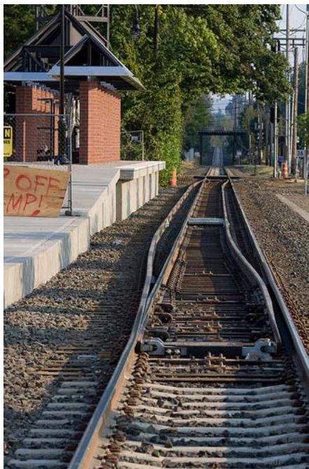
Figure 7-6: Gauntlet track at high-platform station
