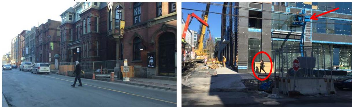
Figure 4 – Without appropriate site controls in place pedestrians are forced to cross streets at unsafe locations or pass directly through an unprotected work area and even underneath active equipment.
