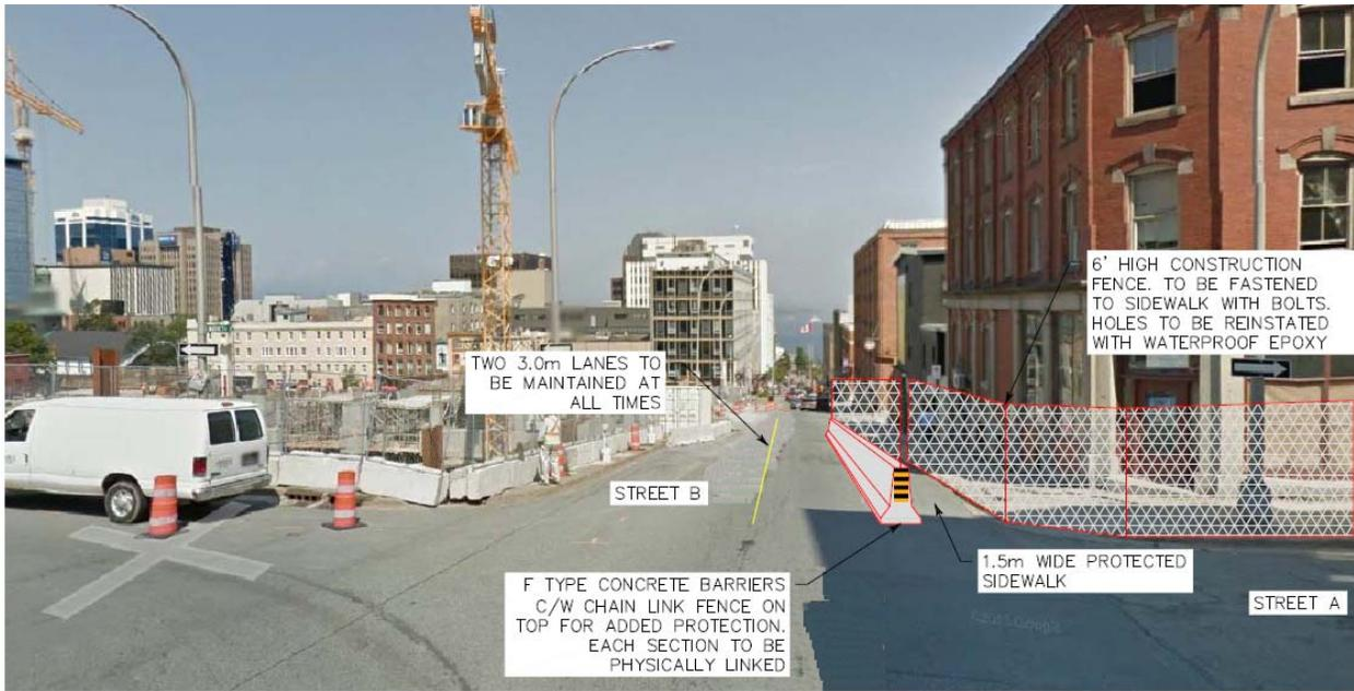
Figure 2 – Proposed protected walkway; Street B. Due to the active construction site on opposite side of Street B, therefore there is no sidewalk on the other side of the street to which direct pedestrians.
