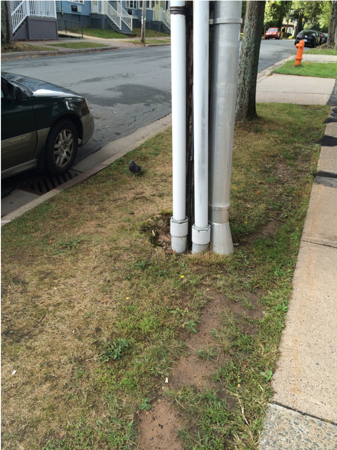
4. Existing utility pole on Henry Street, Halifax (6061 University Avenue)
