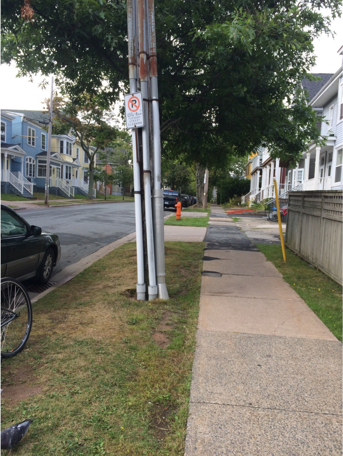
3. Existing utility pole on Henry Street, Halifax (6061 University Avenue)
