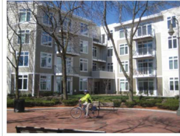
In North Cambridge, Massachusetts, four units are priced below market rate in the 7 Cameron Avenue development, connected by a greenway to bustling Davis Square in Somerville. Credit: City of Cambridge
